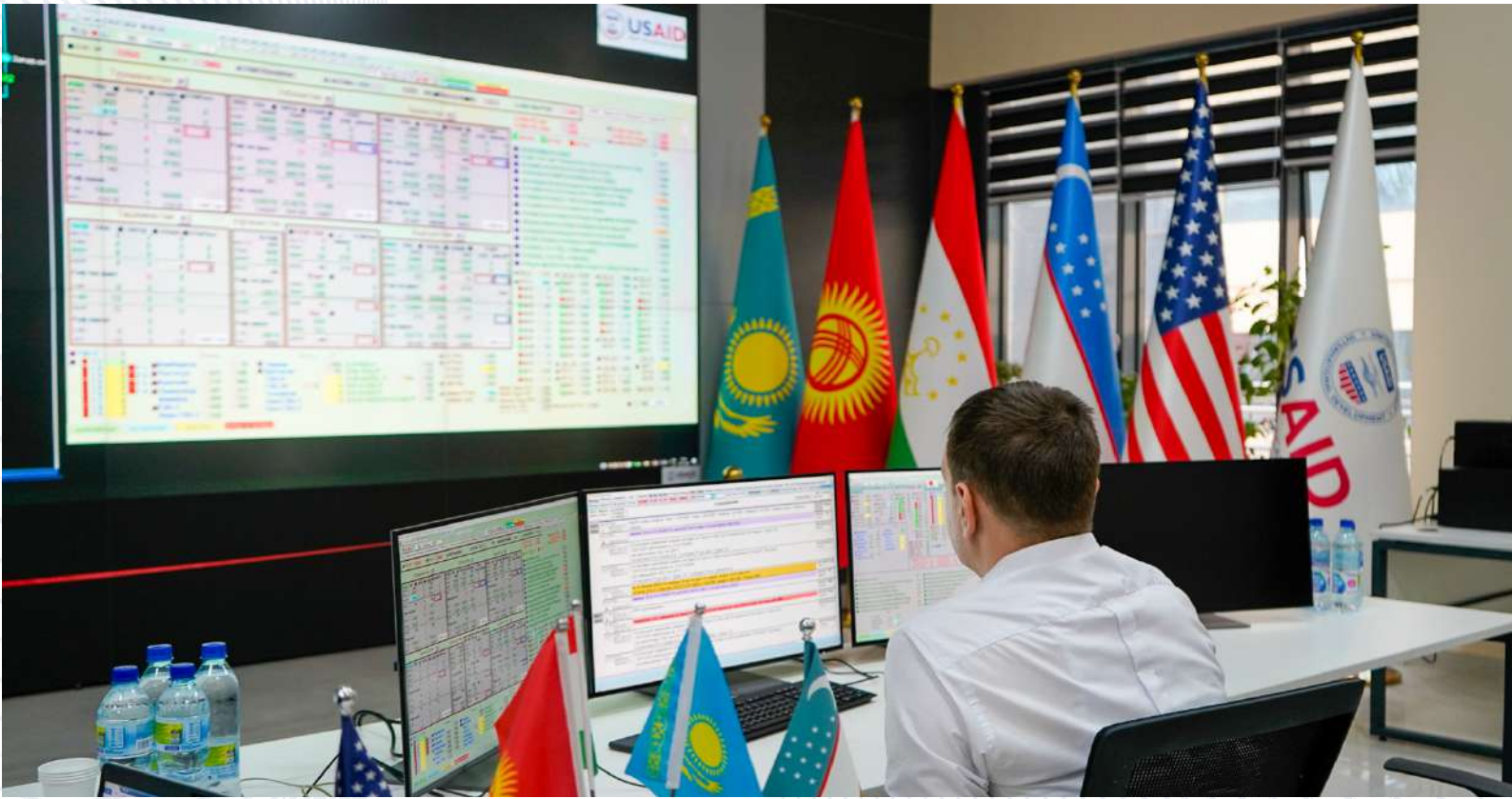
Coordinating Dispatch Center Energia, Tashkent, Uzbekistan
